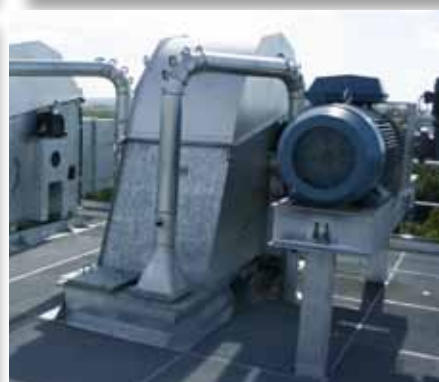
Elevators with discharge suction intakes
